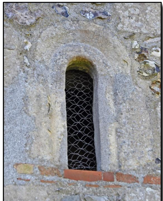
The C15 lights to the stairway have a Norman look to them
