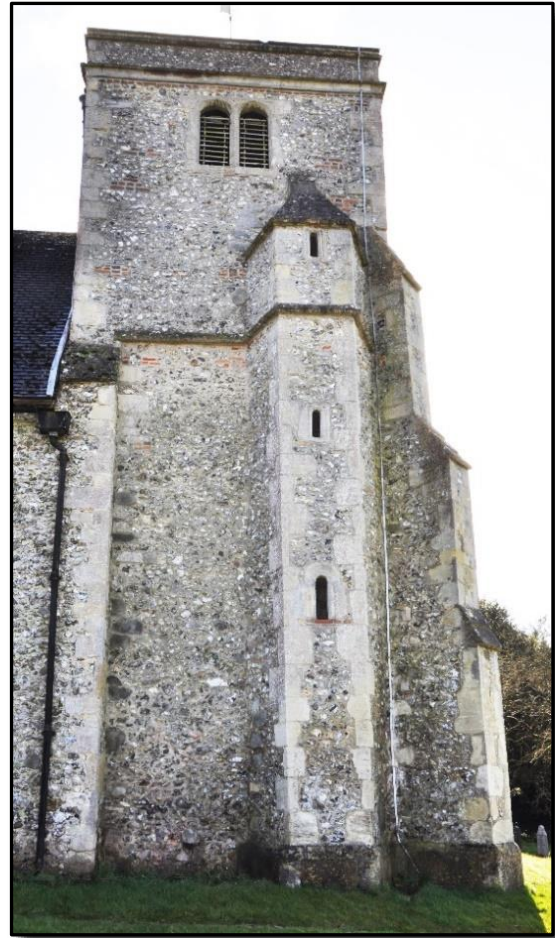
The 2-stage tower with its northern stairway dates from C15.
